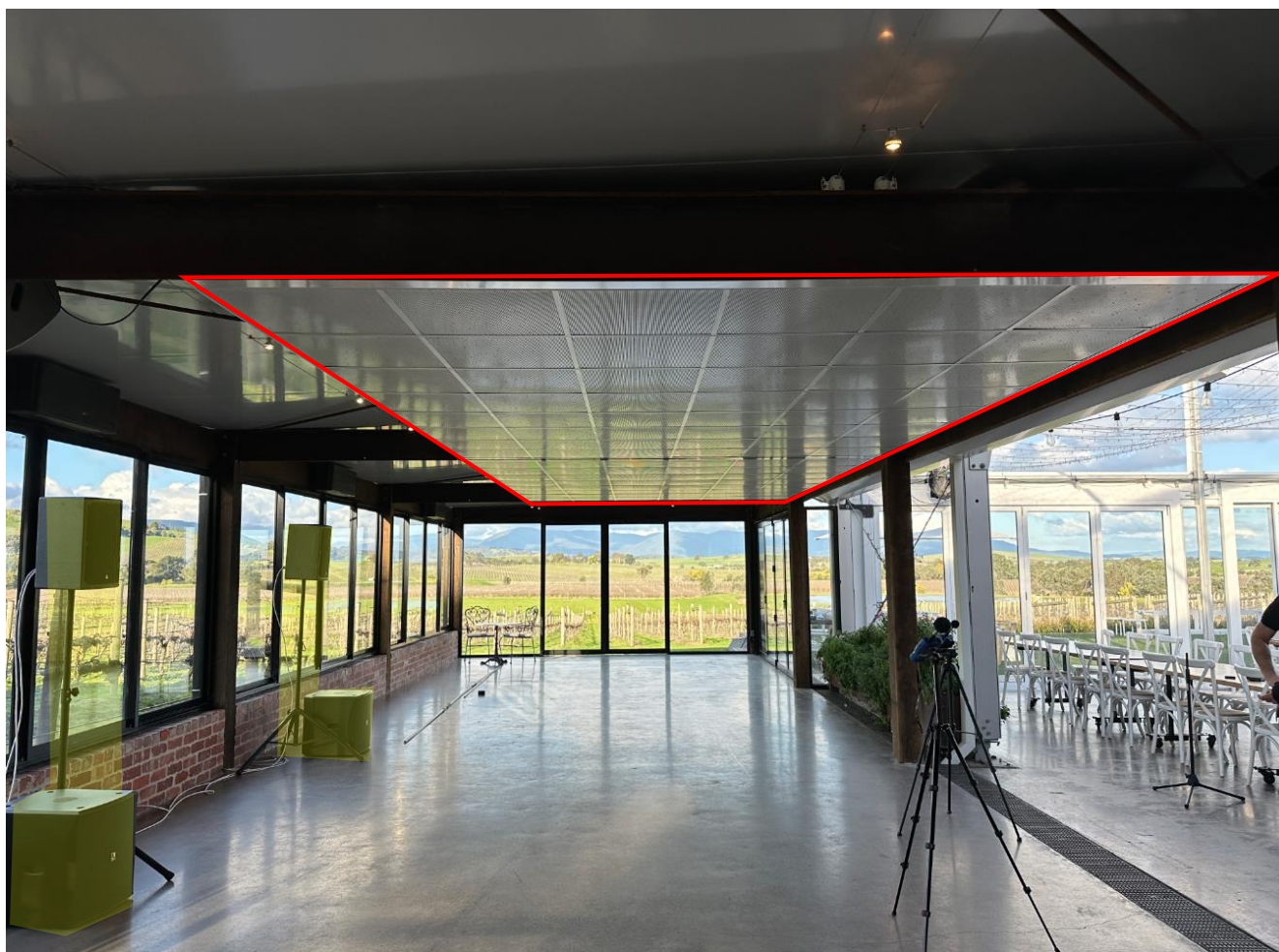
Figure 1 – Installed JBN Sound Ceiling at Acacia Ridge Winery Yarra Valley
